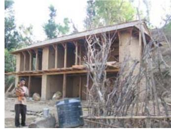
Traditional stone, wood and slate roof houses in Nepali villages use no concrete or steel and cost only \$4000 to build with two stories.
